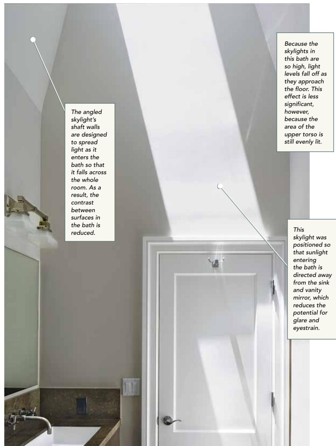
*The angled skylight's shaft walls are designed to spread light as it enters the bath so that it falls across the whole room. As a result, the contrast between surfaces in the bath is reduced.*
